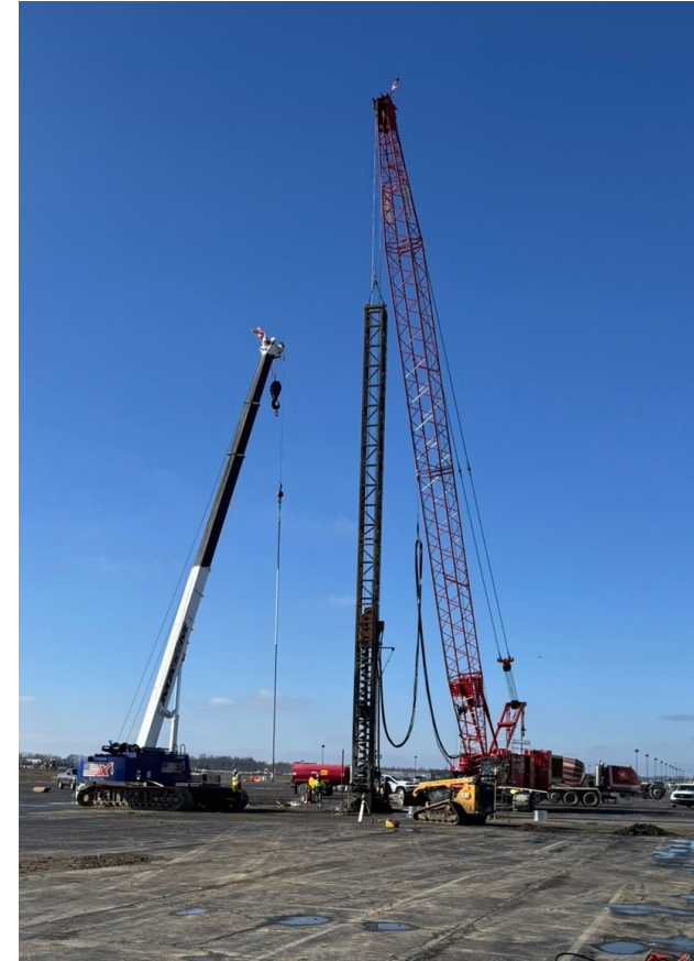
Foundation Test Piles Completed 1-17-25
