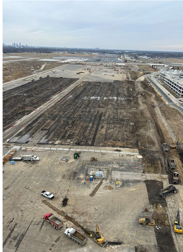
Site Prep/Earthwork Started 1-10-25
