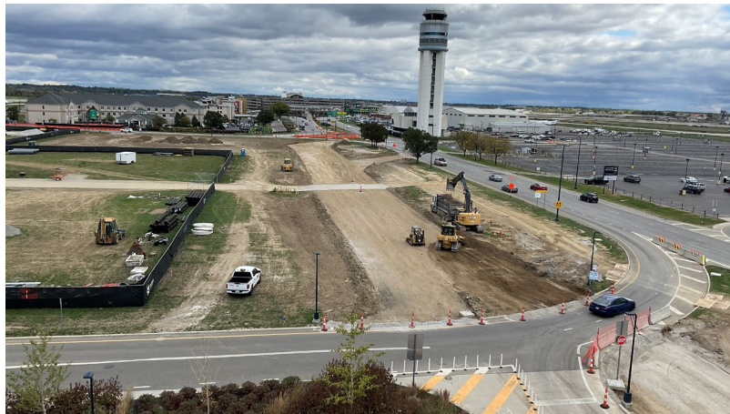
International Gateway Reroute
