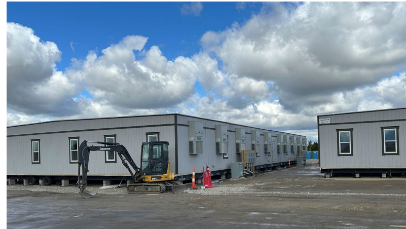
Trailer City Complex
