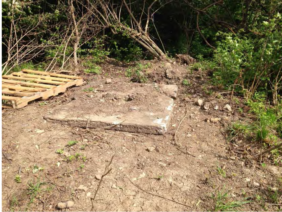
Photo 31. Feature 22, concrete-capped Cistern 2 between the barn and the barn/garage, looking north.
