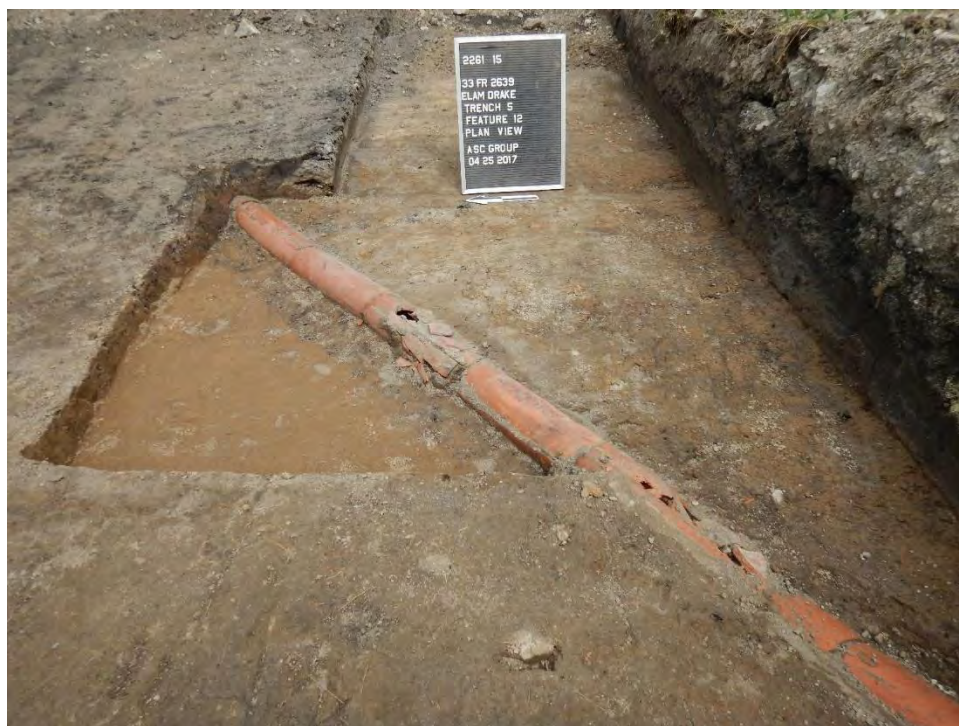
Photo 27. Feature 12, drain pipe identified in Trench 5, looking east.
