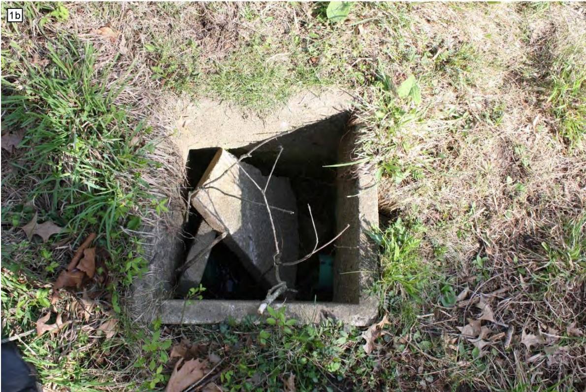
Figure 16. Images of the survey area behind the house, (1a) looking northeast at barn and barn/garage and (1b) looking down at a concrete junction box related to the 20 th century sewer system behind the house.
