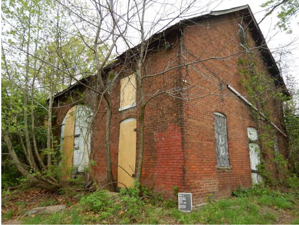
Photo 4. South and east sides of barn, looking northwest.
