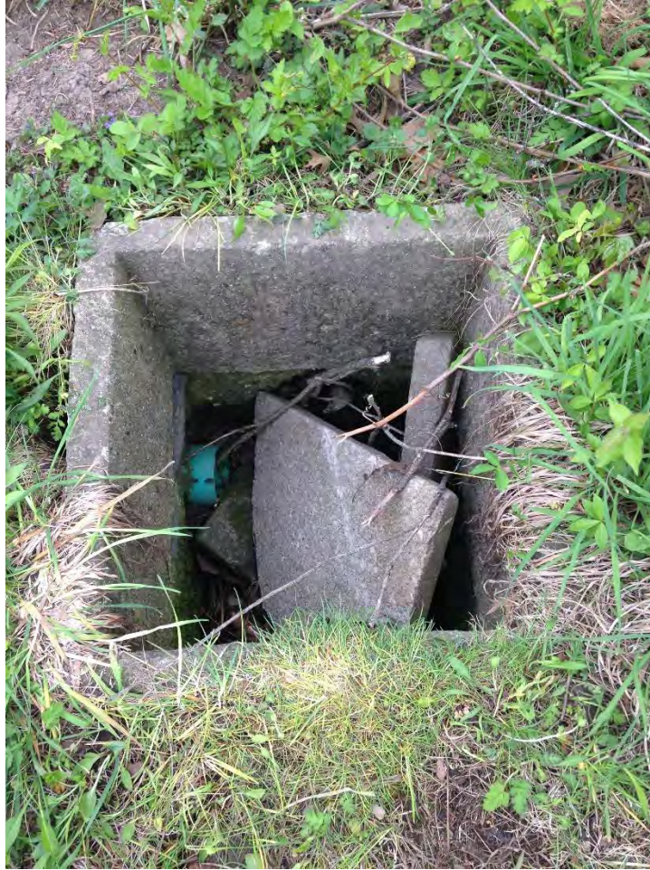
Photo 29. Feature 19, concrete distribution D-box, view north.
