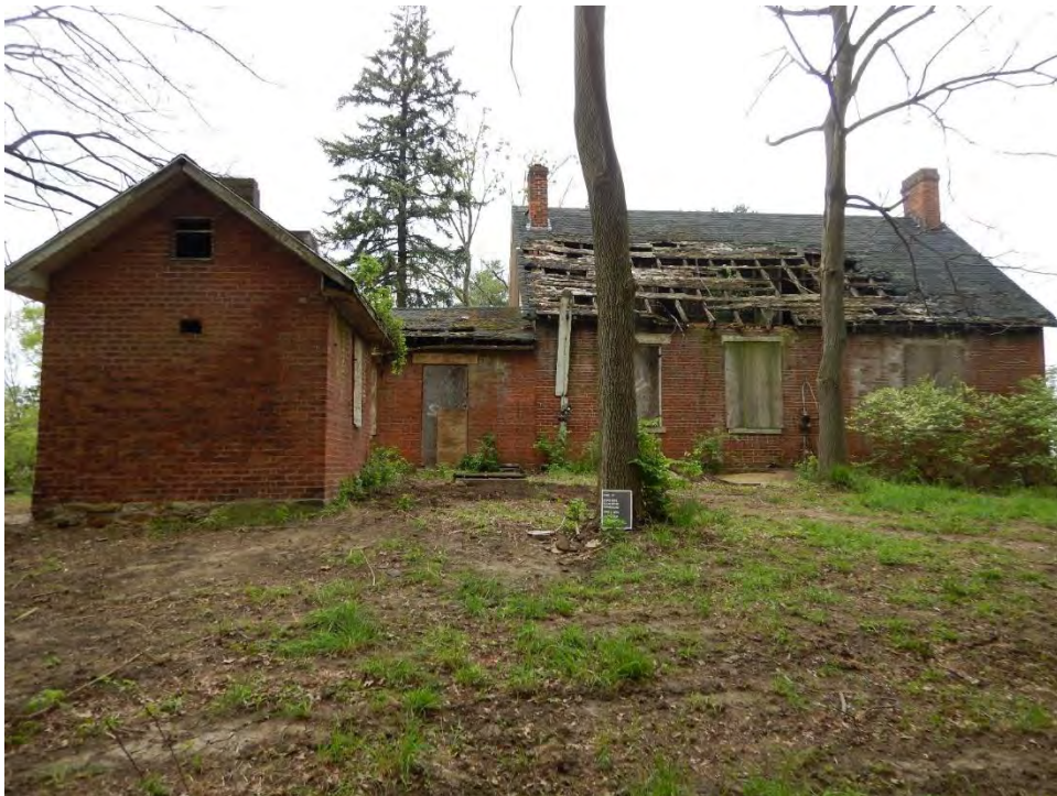
Photo 3. West elevation of smokehouse and house, looking northeast.
